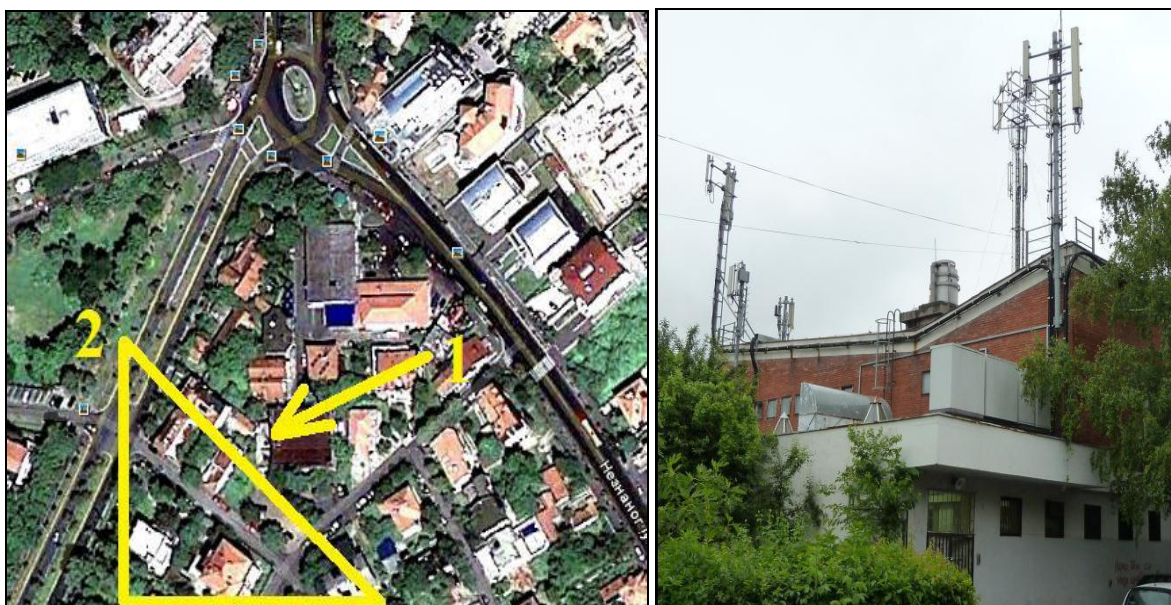
Figure 2. LH side: Marked with 1 is the cooling tower with the fans at the roof of the telephone exchange building; Marked with 2 is the residential area in which SPL caused by cooling fans' noise had to be reduced. RH side: Photo of the telephone exchange building.
