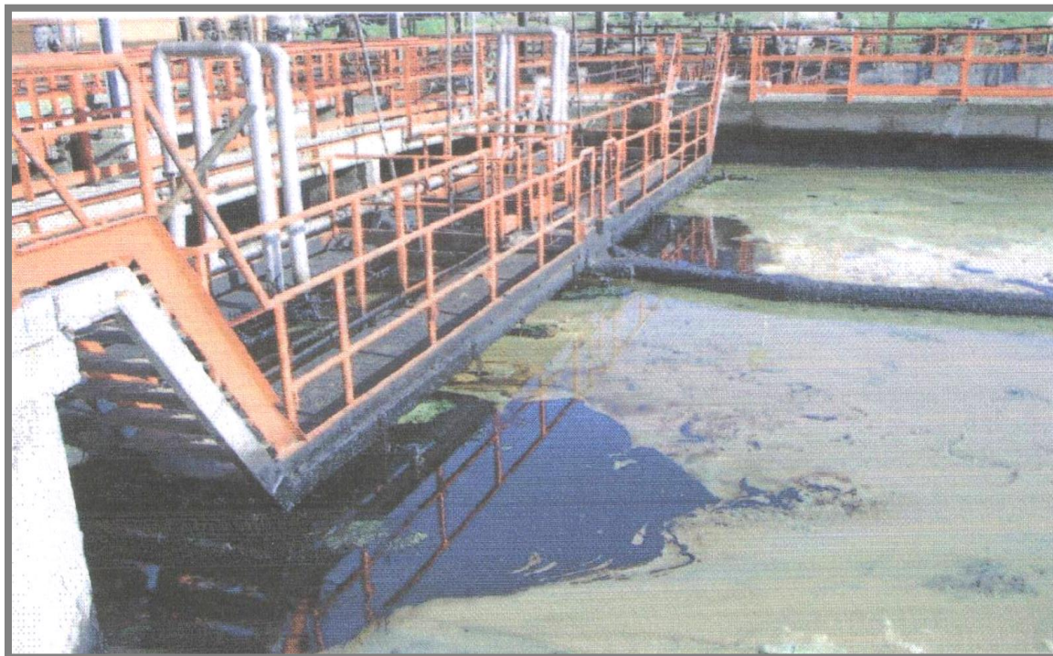
Figure 2. The plant for sedimentation and clarifications of un-oiled water of Petrochemical Refinery in Pančevo
