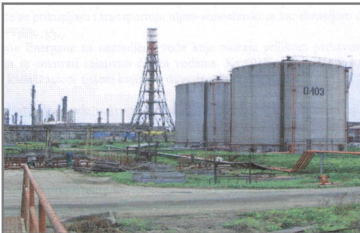
Figure 3. The retention reservoirs
