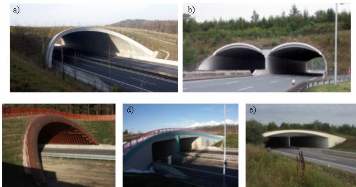
Figure 1. Ecological bridge on highway D11 and motorway R35 in Czech Republic (a), (b), ecological bridge (c) and ecological tunnel on highway D1 (d) in Slovak Republic and ecological bridge on highway A4 (e) in Austria
